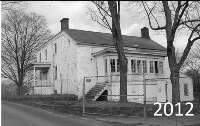
The 1759 Vought House nonprofit took possession in 2012. We have replaced the leaky slate roof with cedar shakes, rebuilt chimneys, removed an enclosed porch and stucco on the front façade, restored windows and the front door. We have begun to restore the decorative plaster ceilings, including the serpent.
