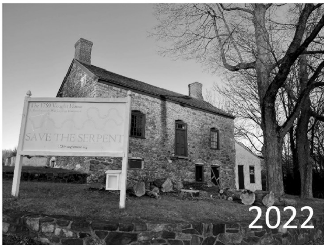
The 1759 Vought House nonprofit took possession in 2012. We have replaced the leaky slate roof with cedar shakes, rebuilt chimneys, removed an enclosed porch and stucco on the front façade, restored windows and the front door. We have begun to restore the decorative plaster ceilings, including the serpent.
